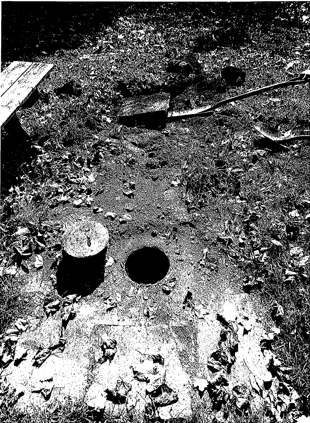
Treatment system 3 septic tank (south) baffle.
