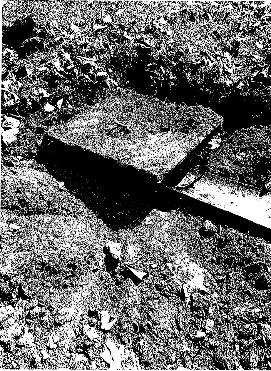
Treatment system 3 septic tank (south) baffle.
