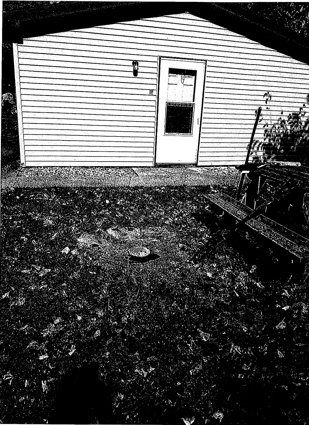
Treatment system 3 Hotel septic tank (South)
