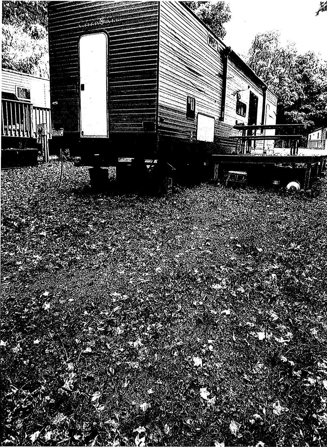
Treatment system 2 Septic Tanks.
